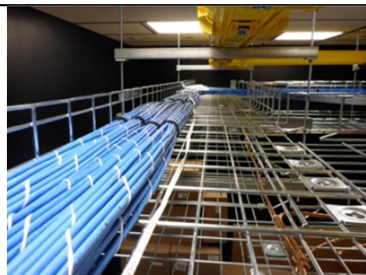
Properly dressed cables in a ceiling mounted cable tray.
