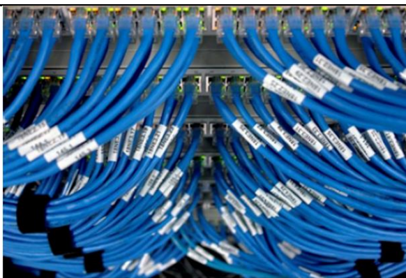
Ethernet patch cables neatly organized and labeled evenly and in-line with machine printed labels
