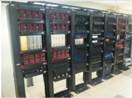
Proper management of patch cables with the use of horizontal and vertical wire managers
